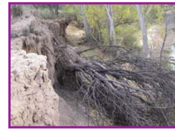
Image 2. Evidence of water erosion of mine tailings adjacent to the San Pedro River, Arizona.
